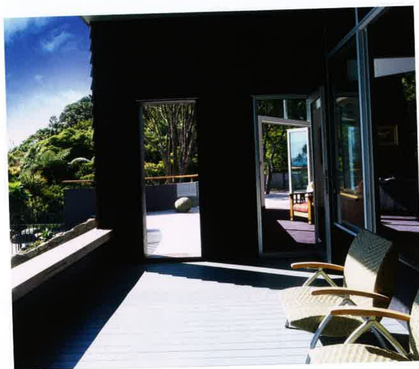
Top: The exterior of the house features black creosote-stained weatherboards—a visual reference to the original cottage on the site. To add interest, the top-floor balcony is clad in alternating strips of copper and macrocarpa.
